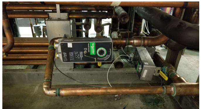
Figure 12: Actuators for Waterside Economizer
