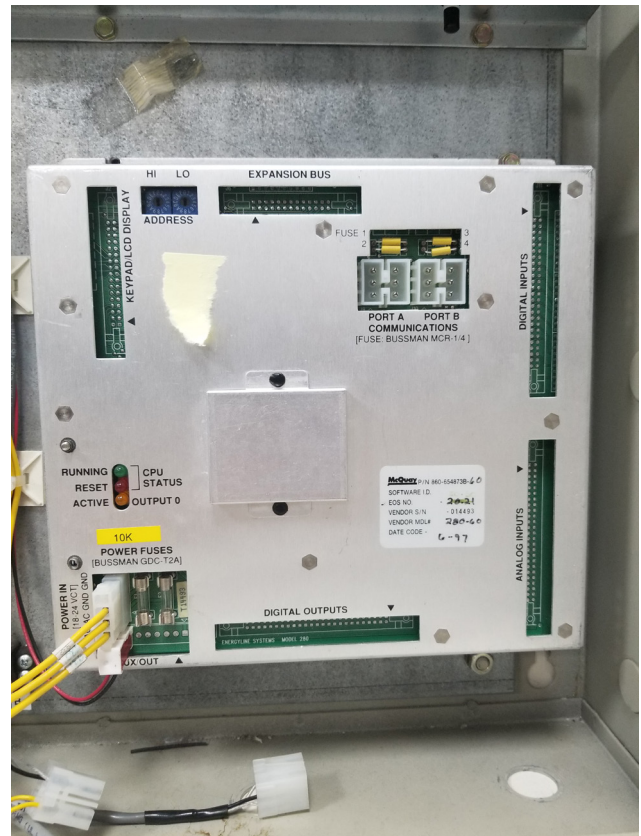
Figure 2: Main Control Board (MCB)
