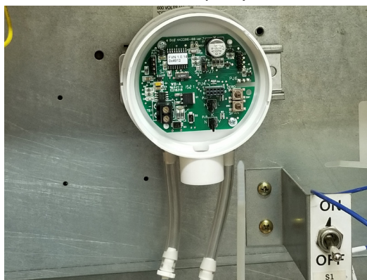
Figure 11: Duct Static Pressure (DSP) Transducer
